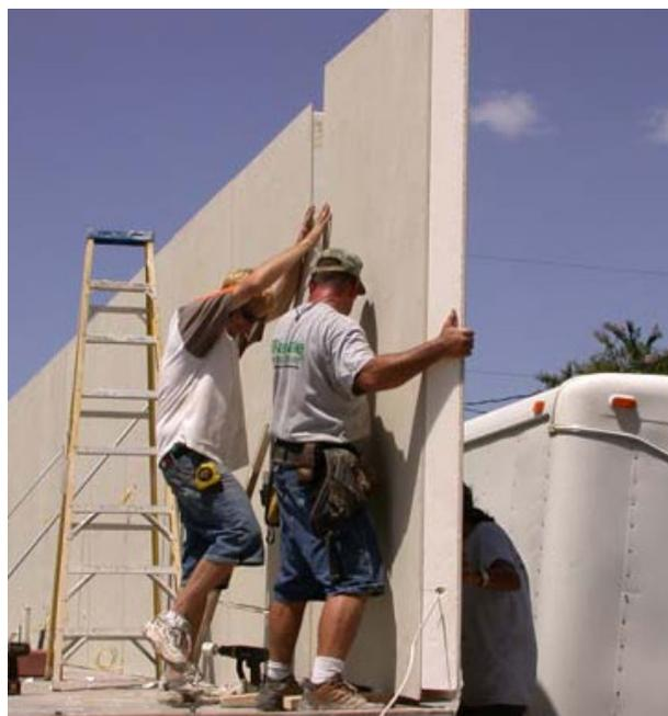
**Figure 8 - CSIP Wall Construction**
