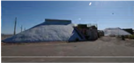
Building 12-63 Constructed in 1969
