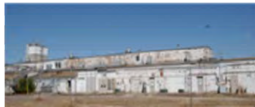
Building 12-21 Constructed in 1945
