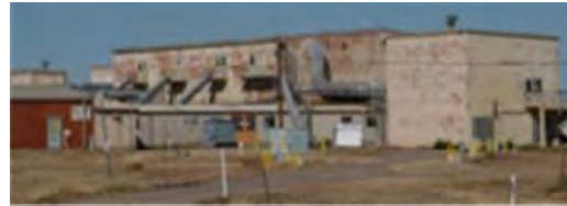
Building 12-17 Constructed in 1945
